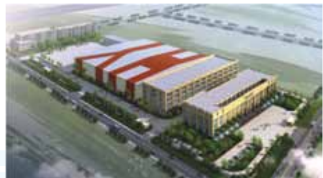
Huayi Plant in Shanghai
